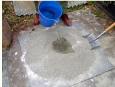
Adding water to refractory concrete
