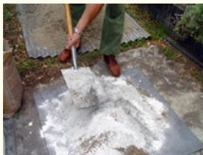
Mixing dry refractory concrete ingredients
