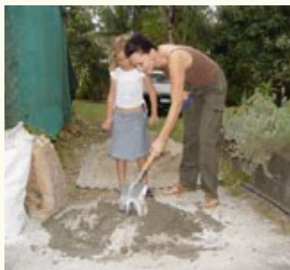
Adding more water to refractory concrete
