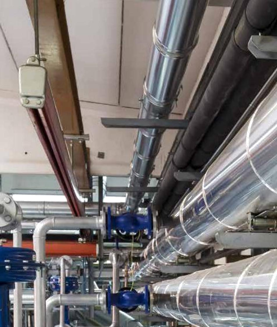
A photograph showing a complex network of industrial pipes and ductwork. Several large pipes are insulated with a clear, flexible foam material called GreenLAG. The pipes are mounted on a steel structure, and various valves, fittings, and sensors are visible. The lighting highlights the metallic surfaces and the texture of the insulation.
